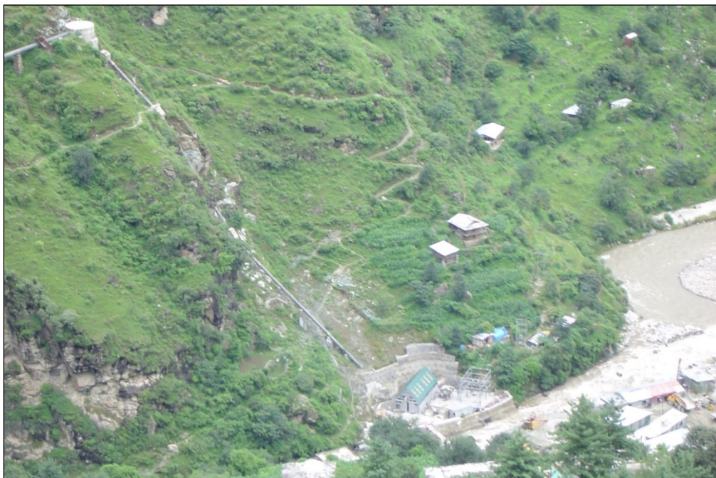
Photo of the Penstock
