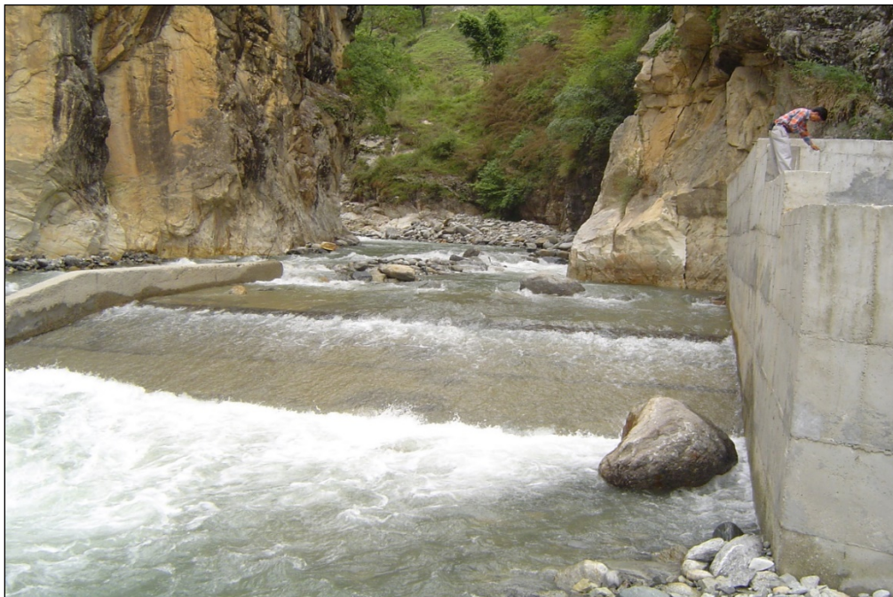
Photo of the Weir Site
