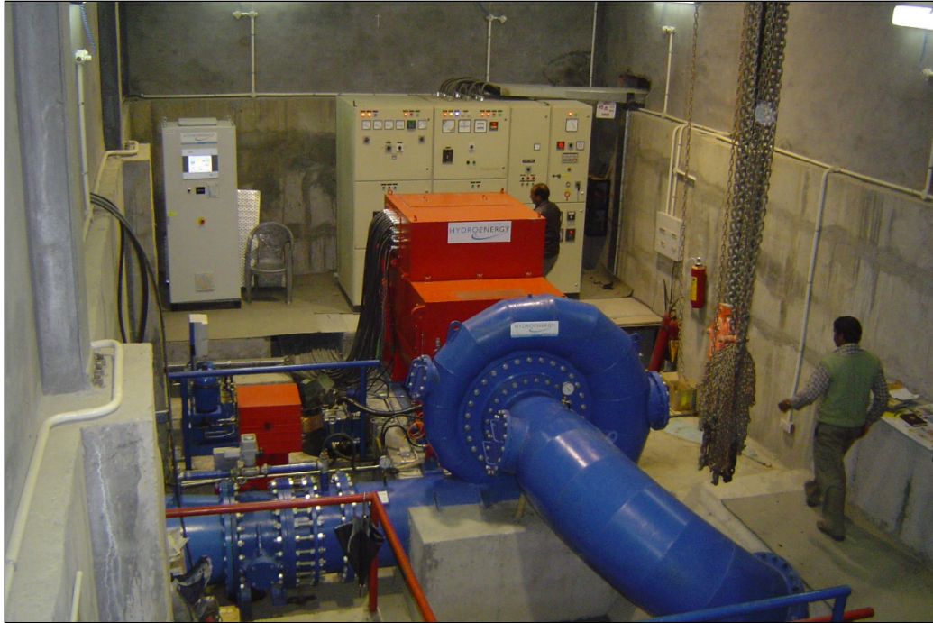
Photo of the powerhouse
