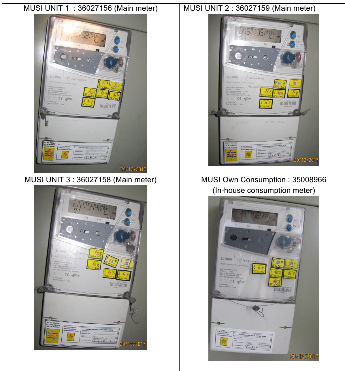
Figure 2 - Picture of main meters main meters and own consumption meter (in-house consumption)
