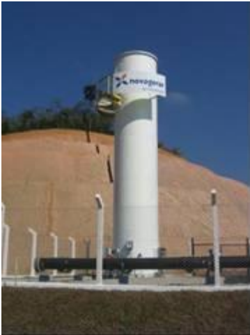
Figure 3 Example of flaring system to be installed. The image above refers to the flaring system implemented on CTR Nova Iguaçu, also operated by Haztec.
