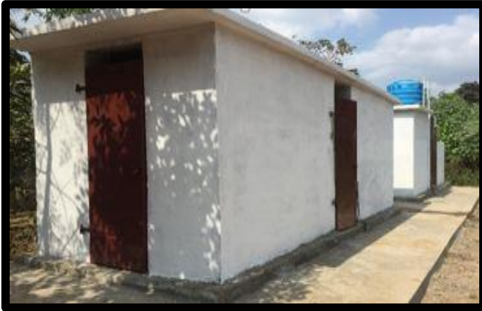
Activity - MPP School Toilets Repairs
