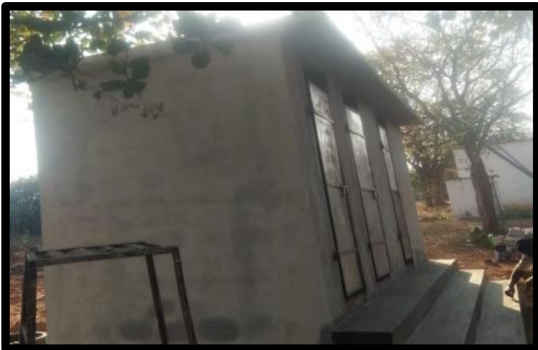
Activity - ZPH School Boys Toilets Construction
