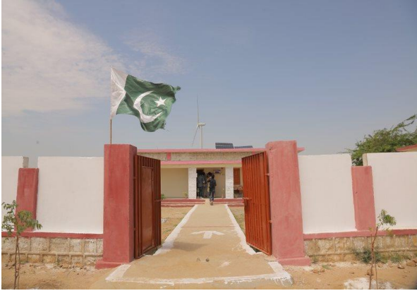
Figure 10: Rehabilitation of nearby school
