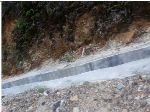
New drainage system in access road near to the power house to minimize the run off
