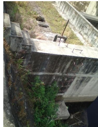
Irrigation sluice in tributary intake 3
