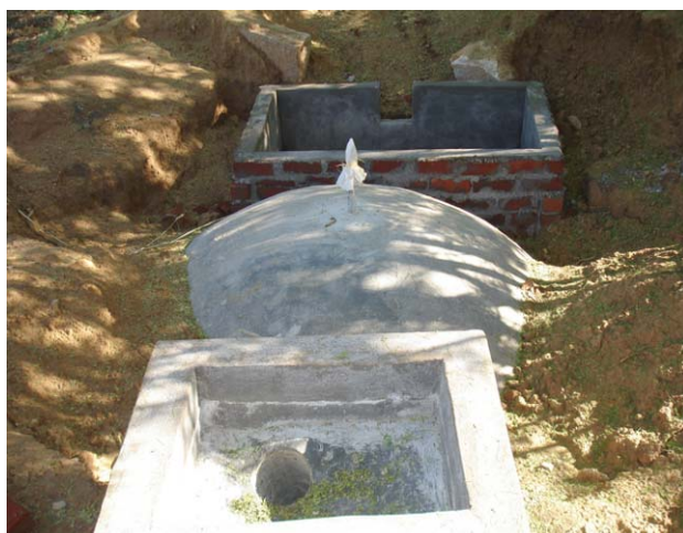
Constructed Deenabandhu Biogas Unit
