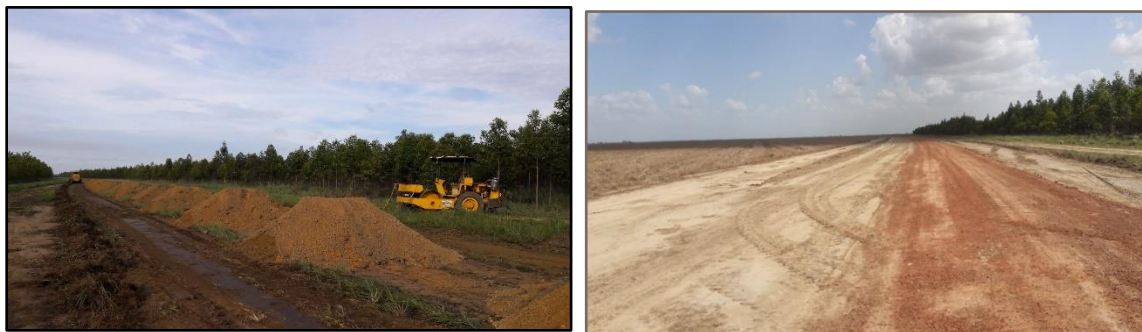
Figure 8: Upgrading of roads
