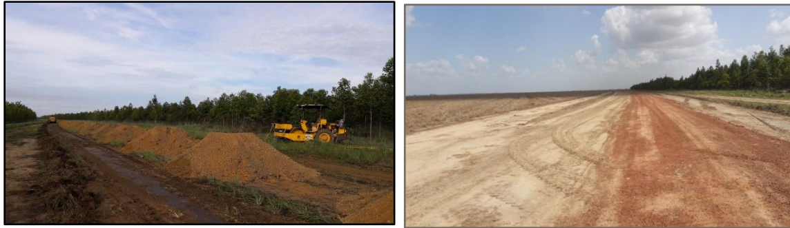
Figure 6: Upgrading of roads
