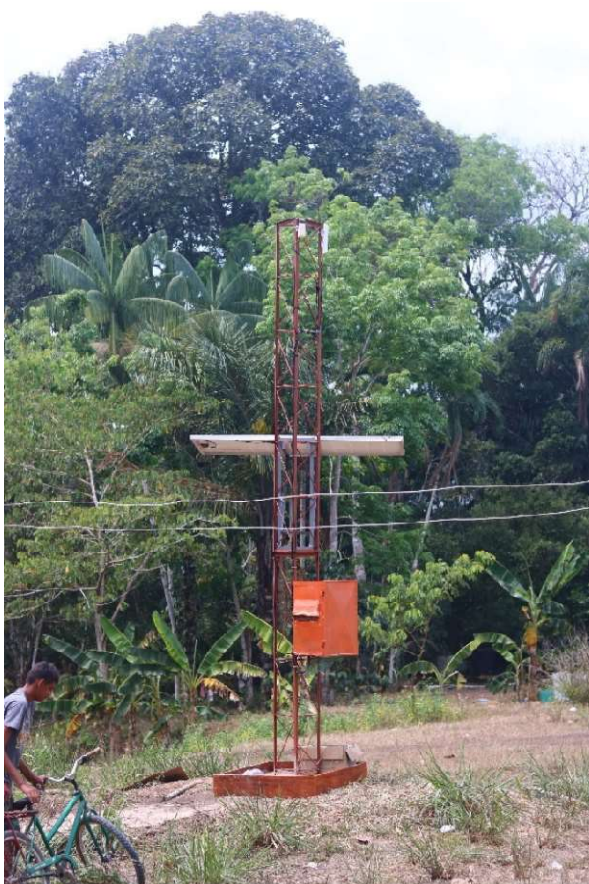
Figure 20: Installation of the internet tower in the Jatuarana community.
