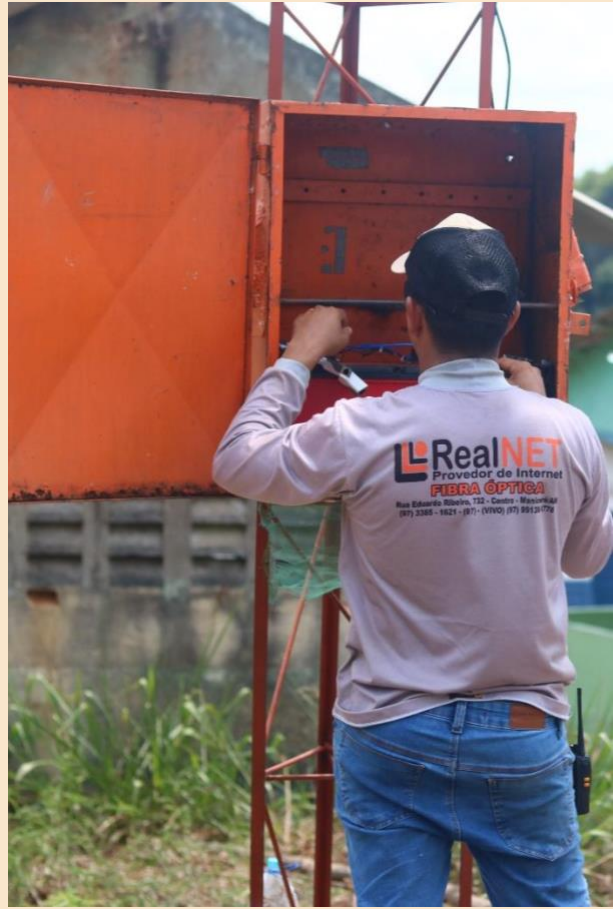
Figure 21: Installation of the internet tower in the Jatuarana community.
