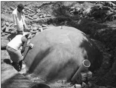
Construction of a biogas Unit
