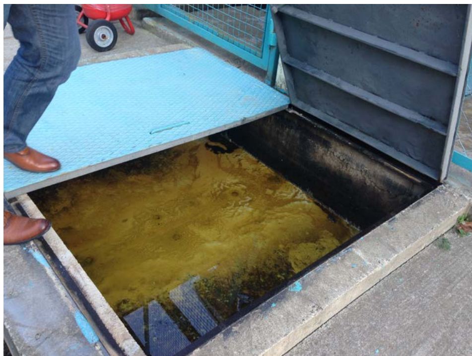
Figure 9:Aralık HEPP Oil drainage system
