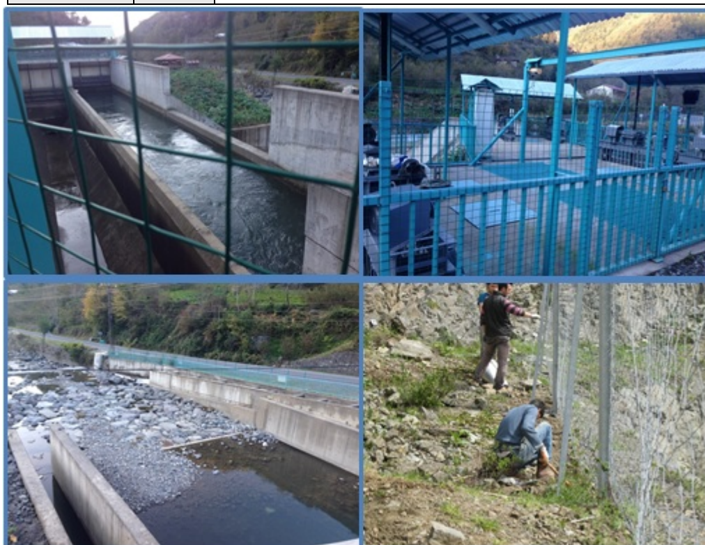
Figure 7: Fencing precautions across the project site
