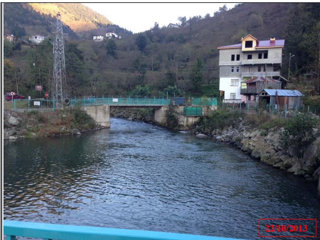
Figure 6. View of reservoir from weir body.
