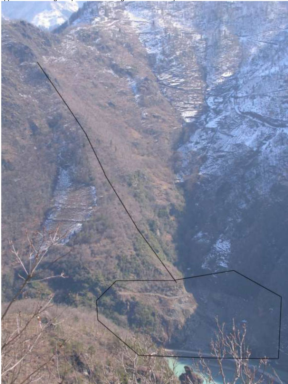
Figure 2. ARALIK HEPP Penstock and Powerhouse Location
