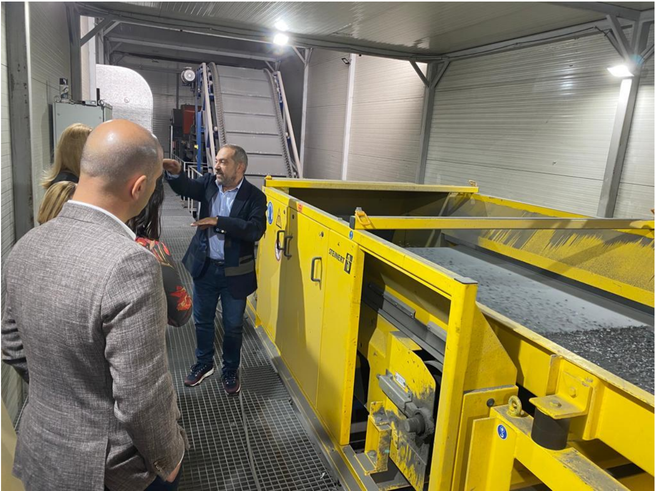
Picture 3. Picture from the visit on the facility site
