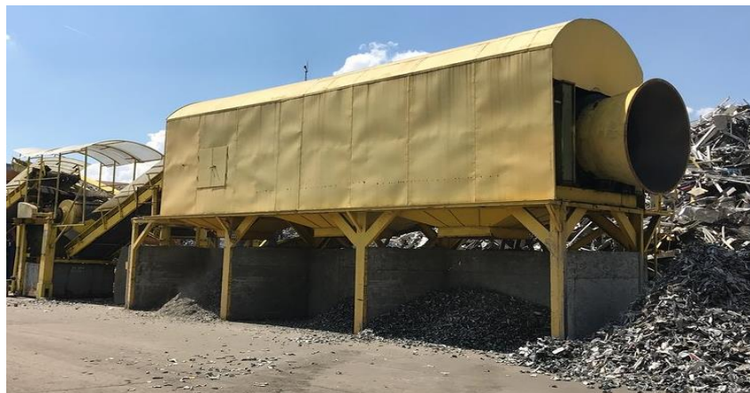
Picture 8: Final fragmentation installation and particle size separation work in progress
