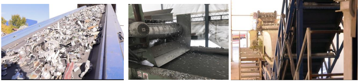
Picture 11, 12 & 13: Conveyor belt, magnetic drum & entire separation installation
