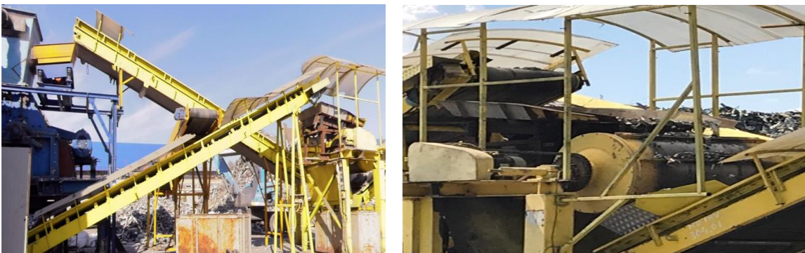
Picture 6 & 7: Final fragmentation installation and electromagnet
