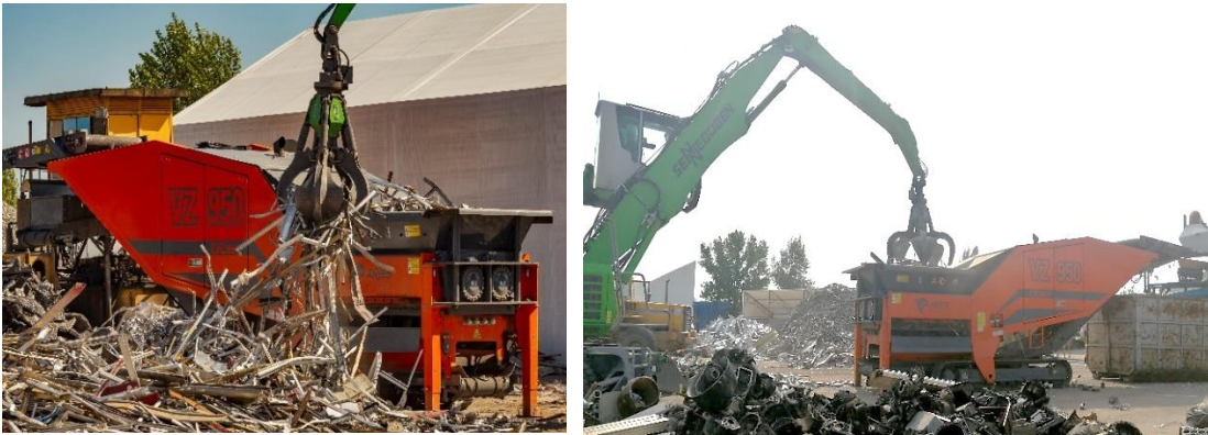
Picture 2 & 3: Loading Arjes machine, Arjes work in progress
