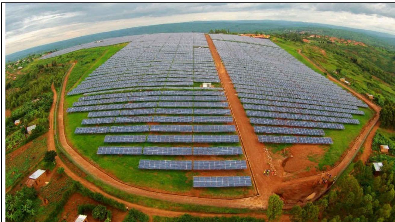
Figure 1: Mounting structure of the CPA
