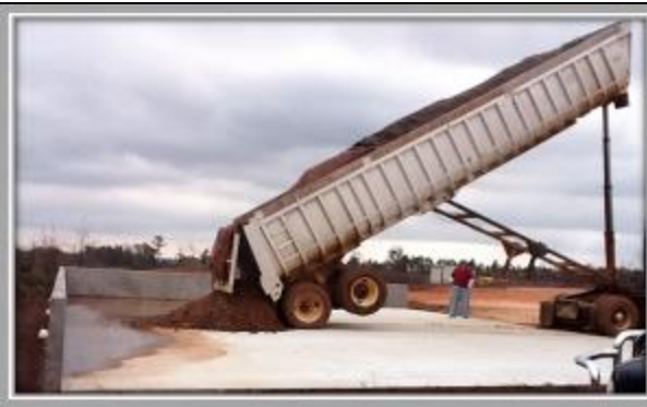
Stage 2: Spreading of waste in cement pad for deodorization
