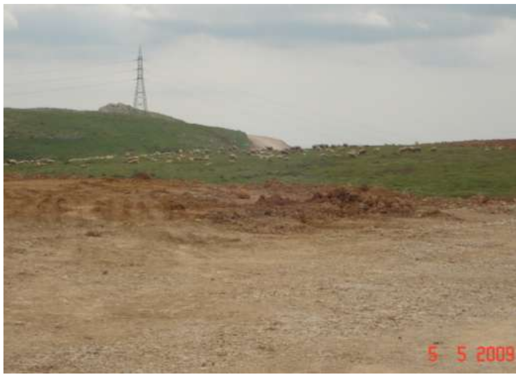
Figure 9. Picture from Ayyildiz WPP construction site
