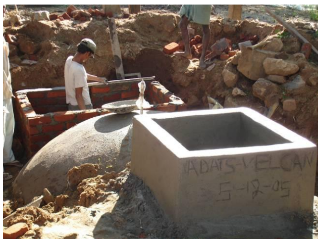
Deenabandhu Biogas Unit in construction
