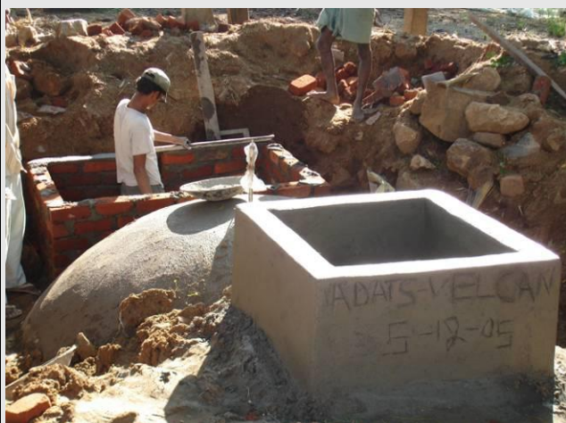
Deenabandhu Biogas Unit in construction
