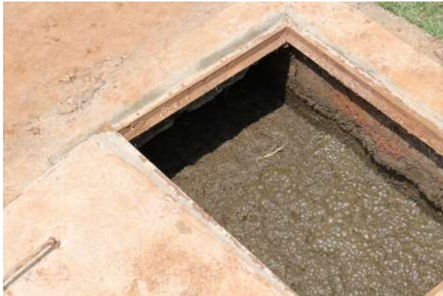
Figure 4: Slurry outlet. Slurry can be applied to agricultural land as a fertilizer.
