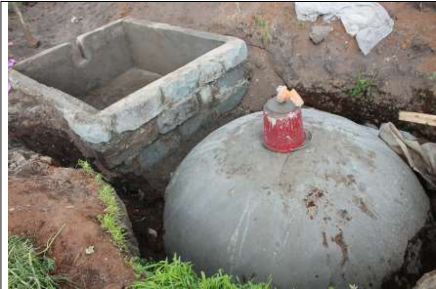
Figure 1: Fixed-dome biogas digester built into the ground
