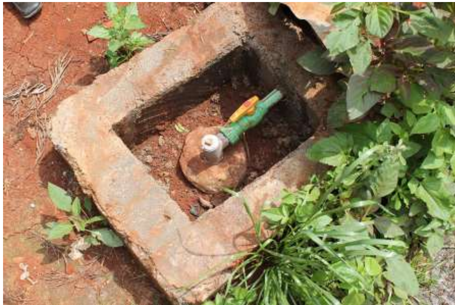
Figure 2: Biogas outlet from which biogas is fed into the household, ready for use
