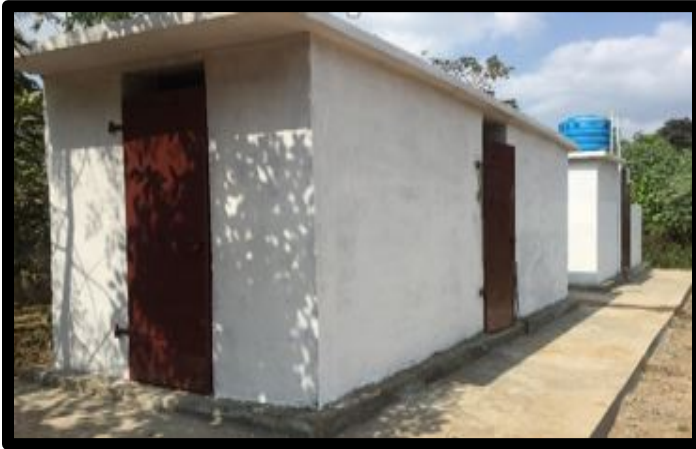
Activity - MPP School Toilets Repairs
