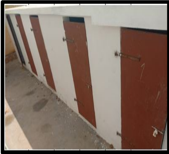
Activity - MPP School Toilets Repairs
