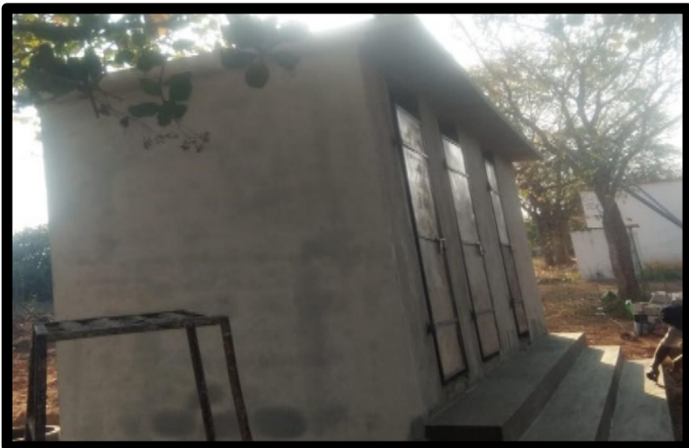
Activity - ZPH School Boys Toilets Construction
