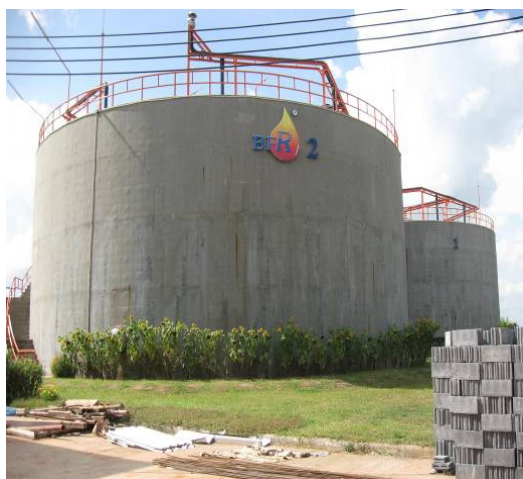
Figure 2. The BFR tanks
