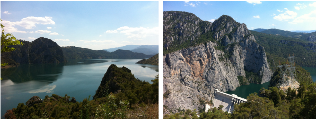
Figure 1 General view of the reservoir lake and general view of the concrete gravity dam.
