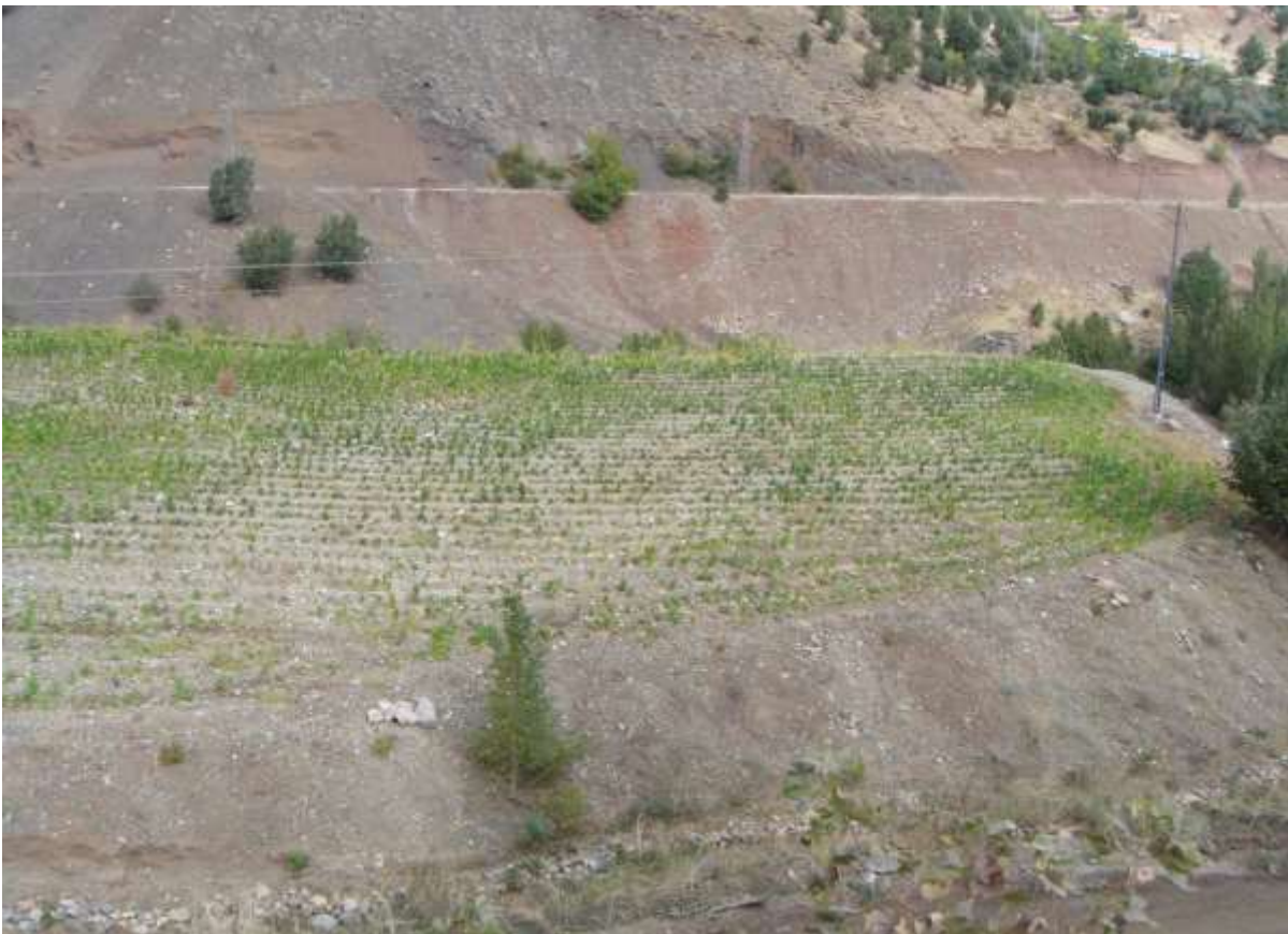
Figure. Proper storage and use of aggregates from excavation Works at the Project site. Planting trees helps to take precautions against erosion problem
