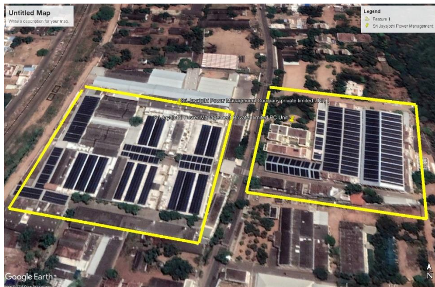
Figure 5 -Google Earth Image of Sri Jayajothi Power Management Company Private Limited UNIT I & PC UNIT
