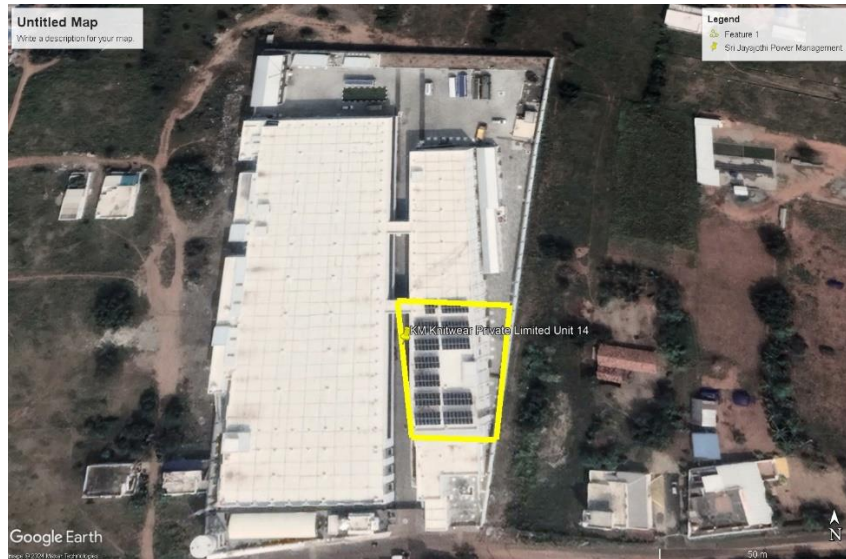
Figure 4- Google Earth Image of KM Unit 14
