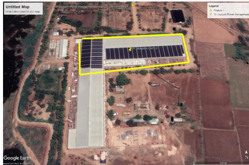
Figure 6- Google Earth Image of Sri Jayajothi Power Management Company Private Limited UNIT II
