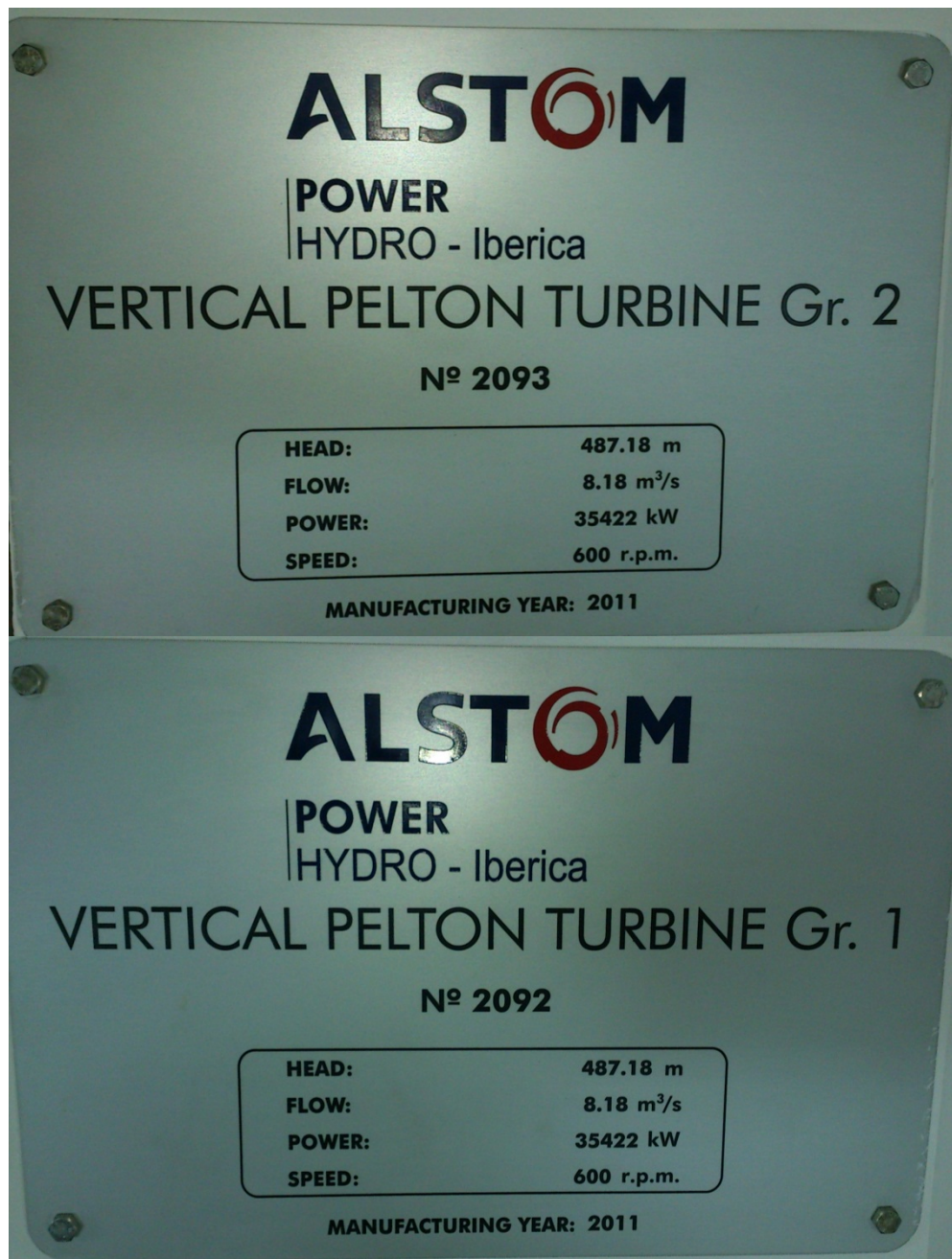
Figure 2: Nameplates of the 2 turbines installed at Büyükdüz HEPP
