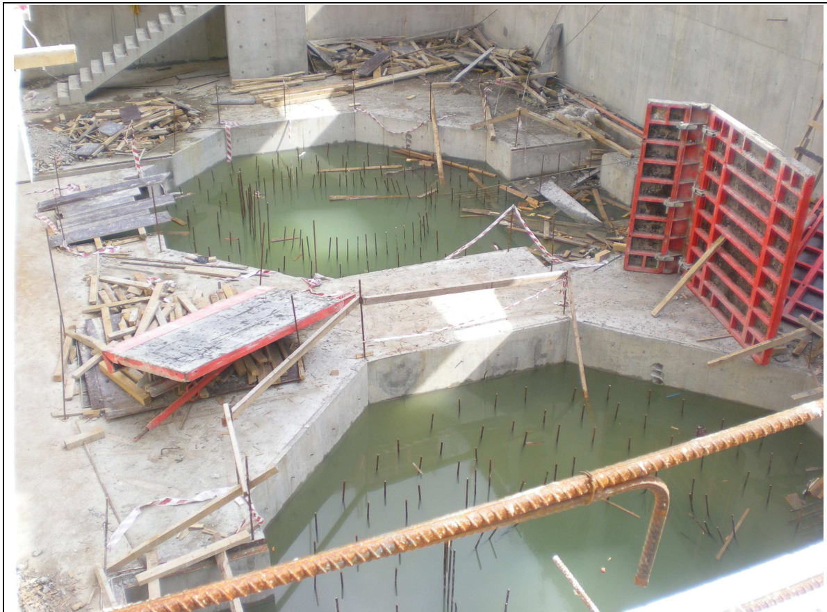
Photo 3: Project Powerhouse Construction
