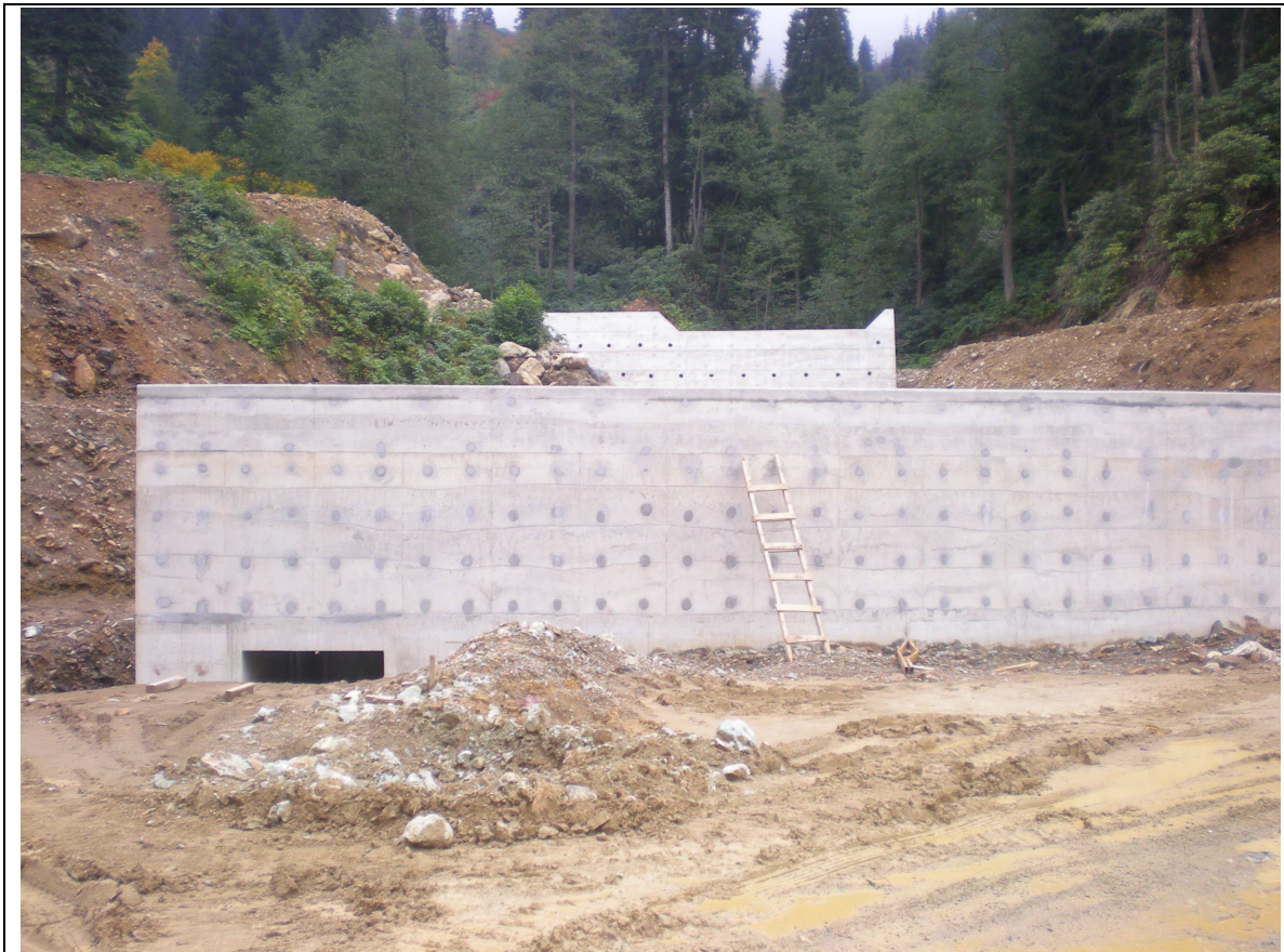
Photo 2 : Project Weir Construction
