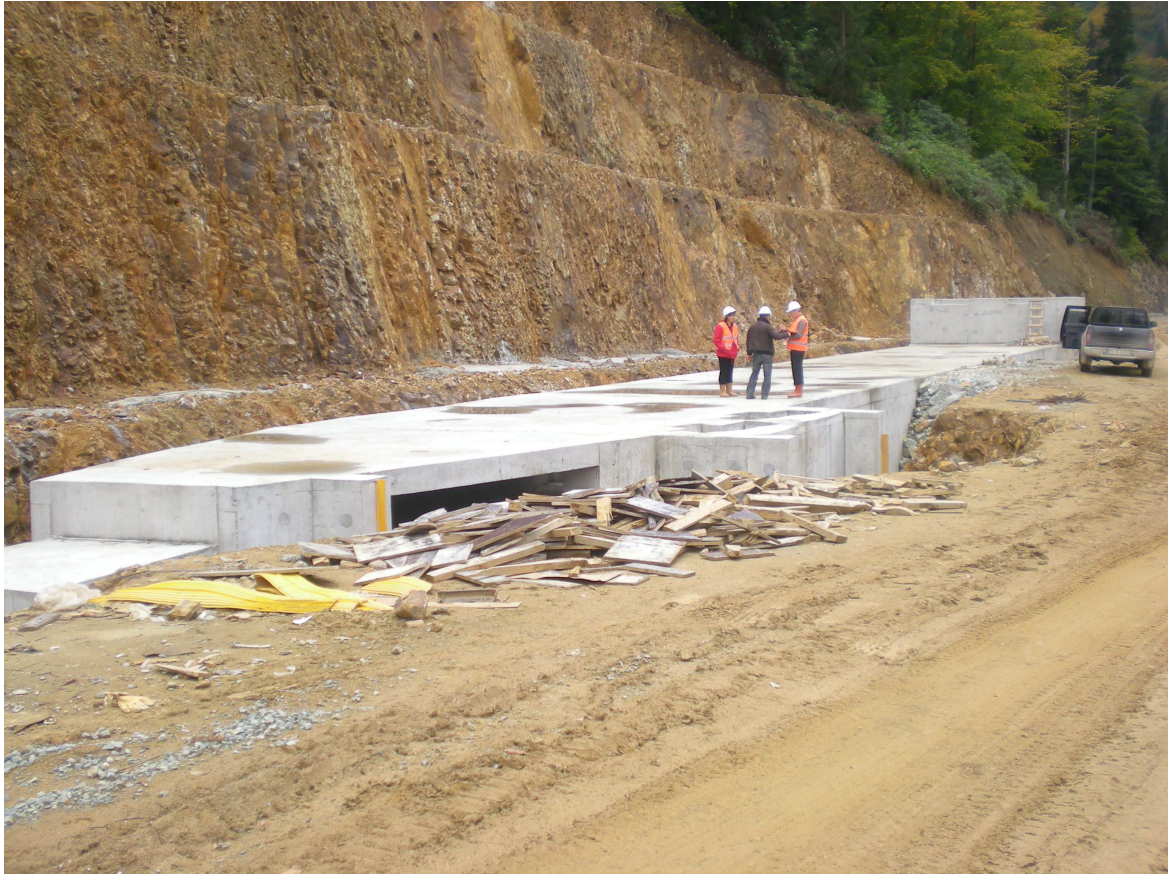
Photo 1: Project Weir Construction
