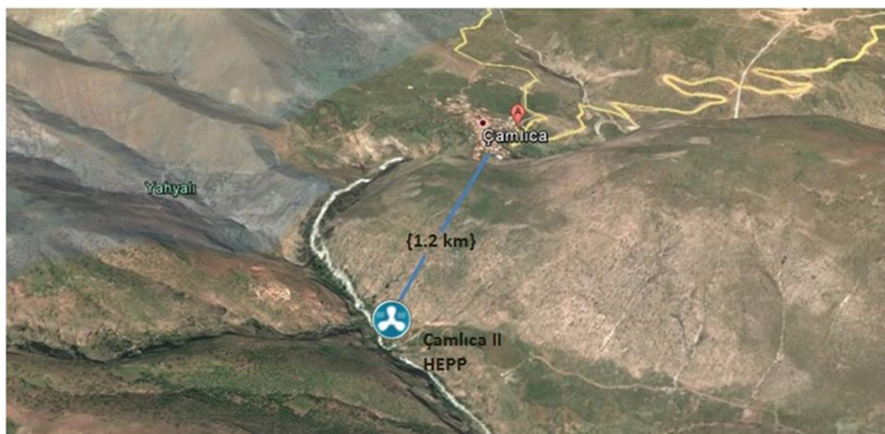
Figure 1. Çamlıca II HEPP project site
