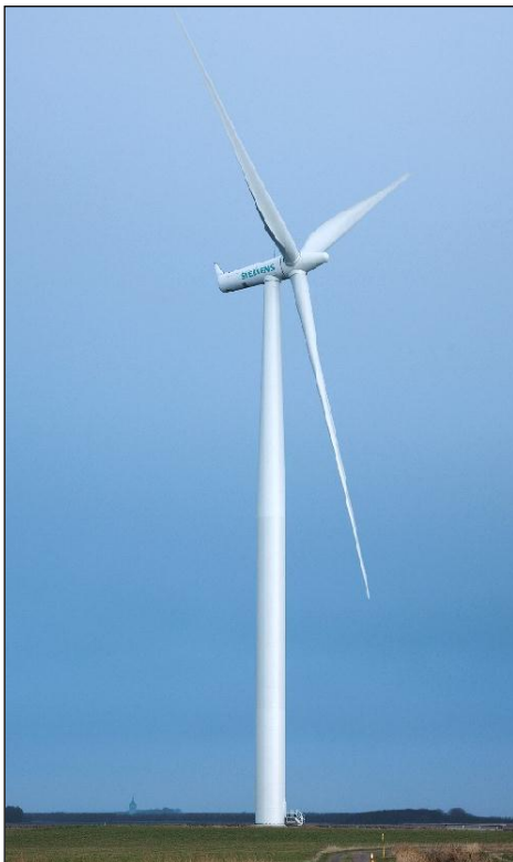
Figure.1. View of Siemens SWT 101
