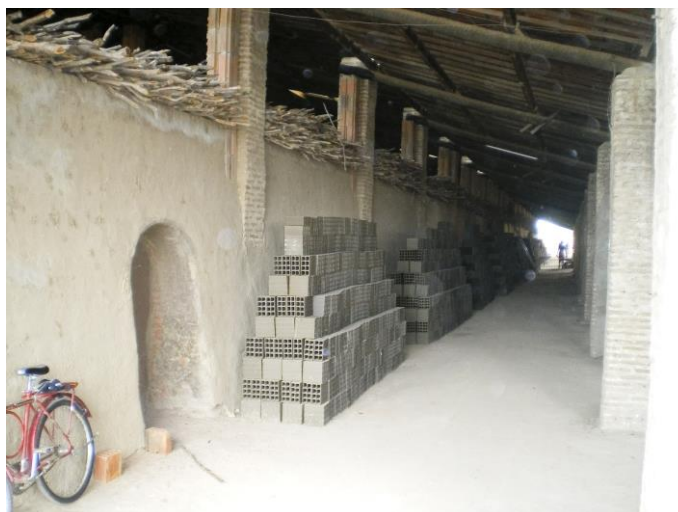
Figure 05. Hoffmann kiln being fed with renewable biomass in Santa Rita Ceramic.
