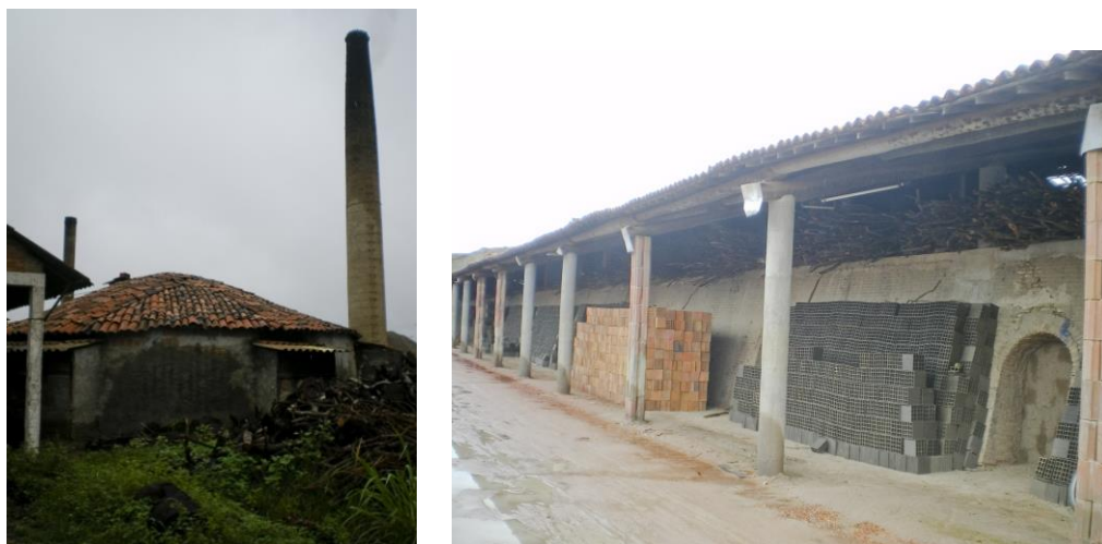
Figure 02. Round and Hoffman kilns at Ceará Ceramic.
