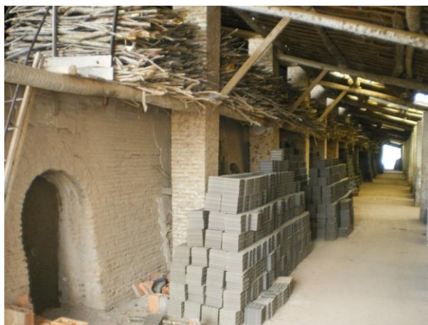
Figure 01. Hoffmann kiln being fed with renewable biomass in Antônio Ceramic.
