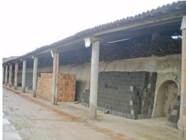
Figure 4. Hoffmann kiln being fed with renewable biomass in Ceará Ceramic.
