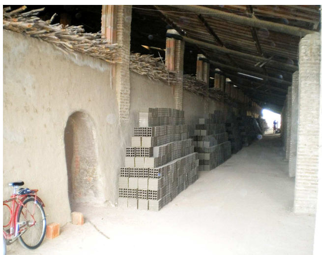
Figure 06. Hoffmann kiln being fed with renewable biomass in Santa Rita Ceramic.
