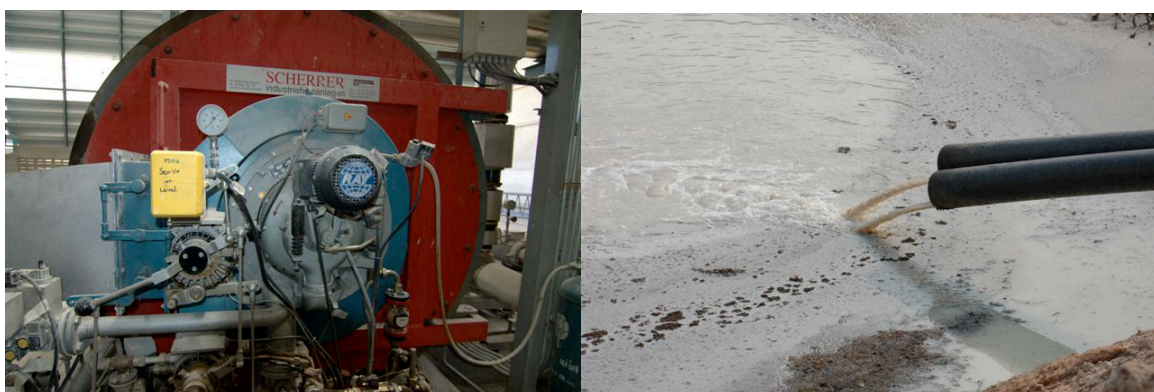
Figure: Pictures of thermal oil boiler that will use biogas plus existing wastewater treatment lagoon system
