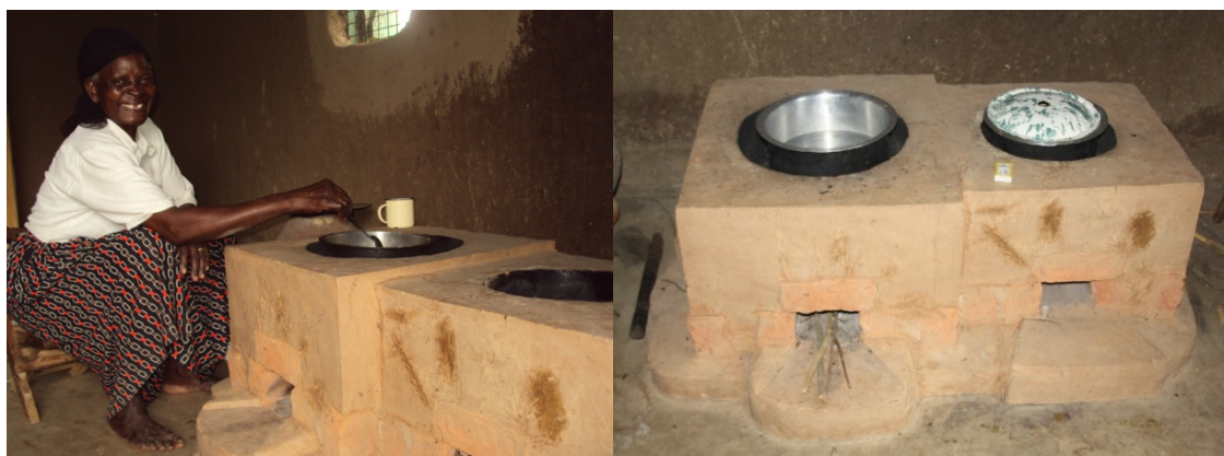
Installed project rocket stove with two cooking units.
