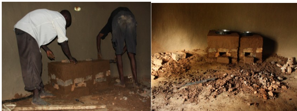
Fig 15 & 16: Adding bricks and mud to give the stove its final shape
