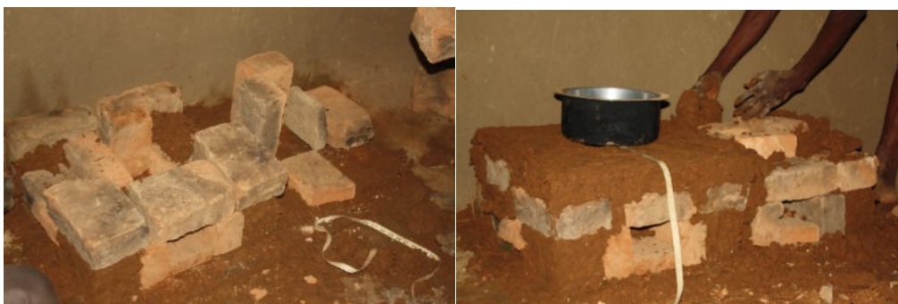
Fig 13: & 14: Arranging brick for the combustion chamber using measuring tapes and pots
