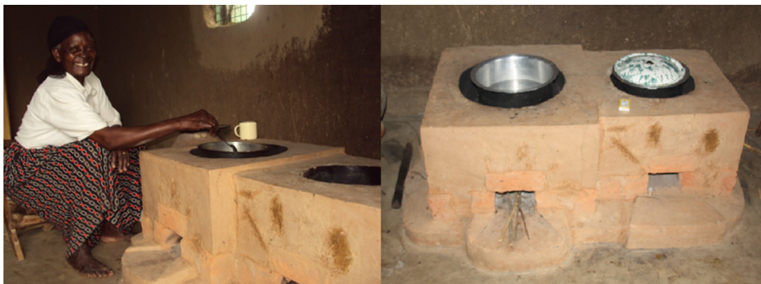
Fig 10: Installed, ready for use, project rocket stoves with two cooking units.
