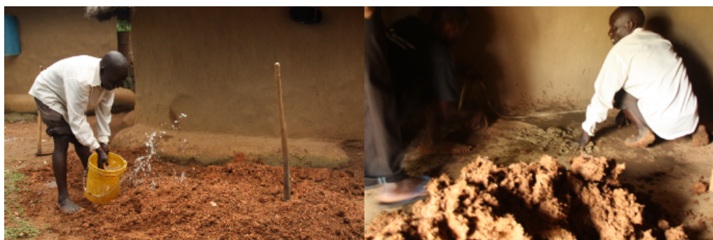
Fig 11: Mixing materials (mud and sawdust) Fig 12: Preparing stove location
