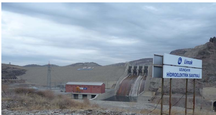
Figure 1: Hydropower Plant, 8 th December 2011
