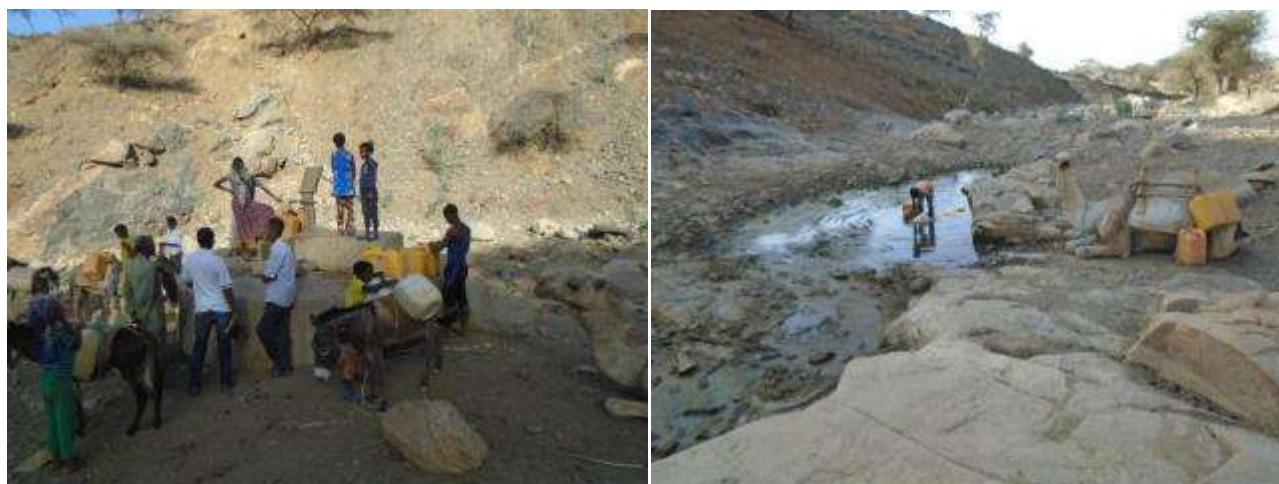
Pic.4 Water Source in Dighibeofre and after boreholerehabilitation
