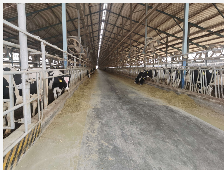
During onsite investigation, it was verified feed is intensively
