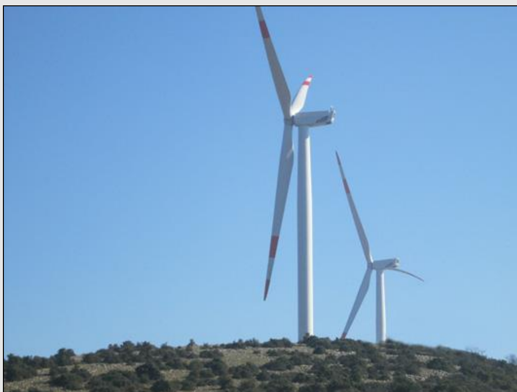
Figure 6 The picture of turbines at Kayaduzu WPP
