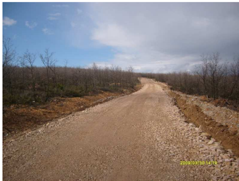
Road fill works
