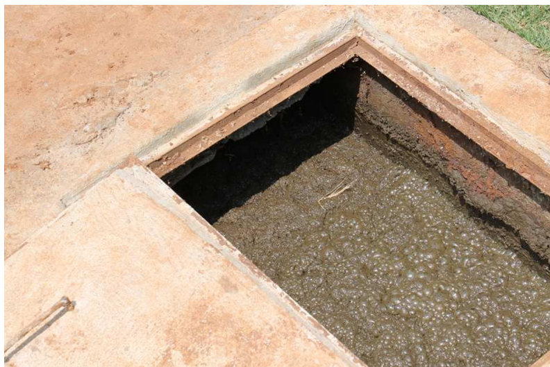
Figure 4: Slurry outlet. Slurry can be applied to agricultural land as a fertilizer.
