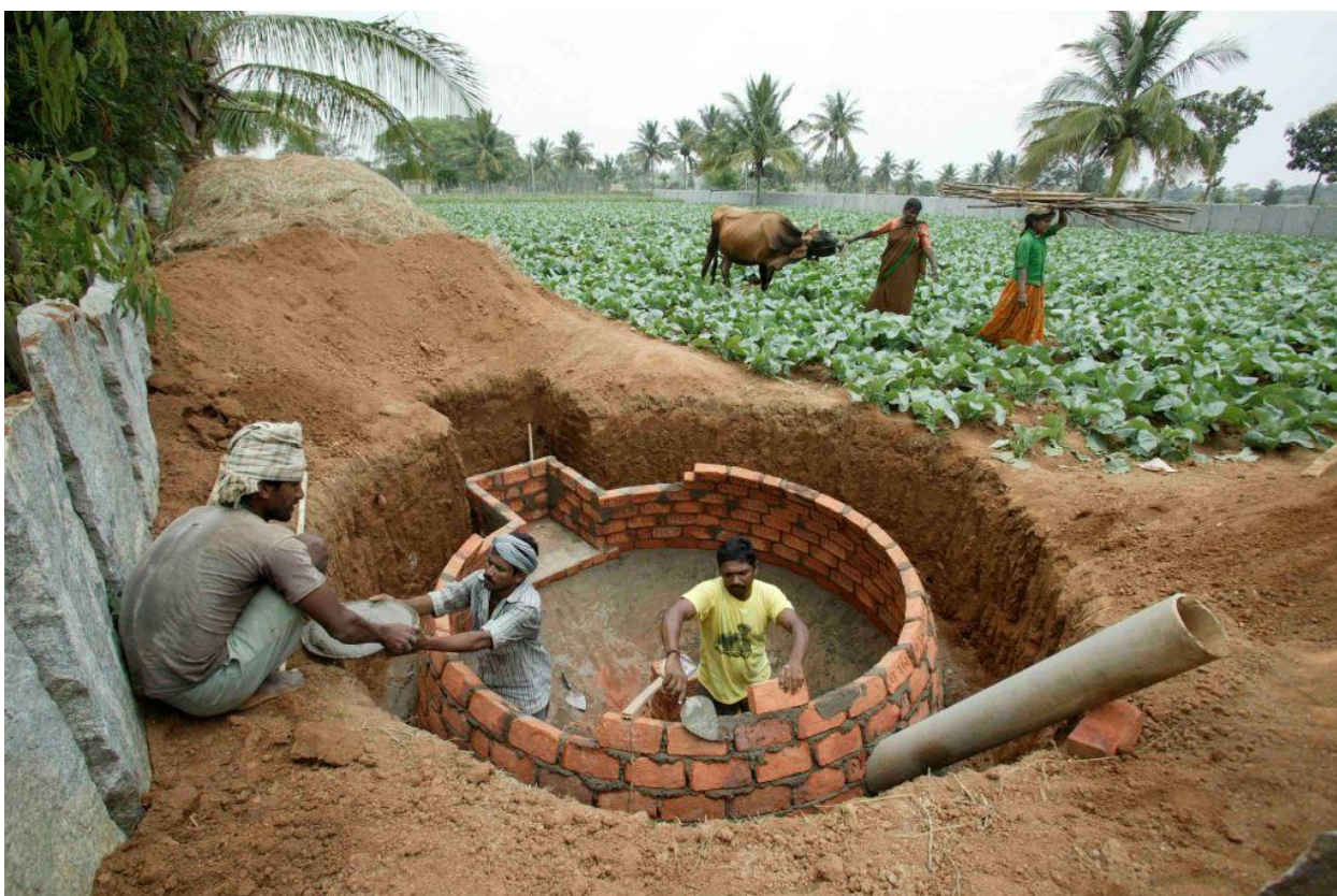
Biogas digester under construction
