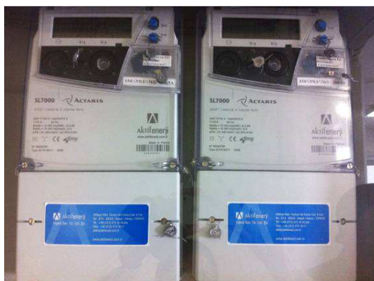
Figure: Meters sealed and used by TEİAŞ for taking monthly readings
