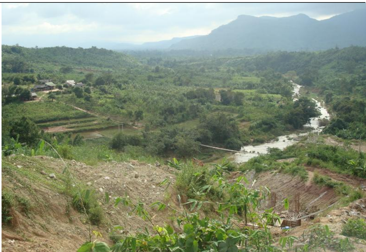
Figure 1: View along the future penstock fundement towards powerhouse and La La River (Picture during construction)
