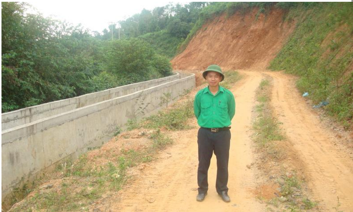
Figure 3: Water channel bringing water from the dam to the penstock
