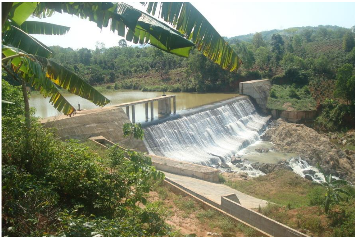
Figure 2: Small Dam of the La La Hydropower Plant, afforestation in the back
