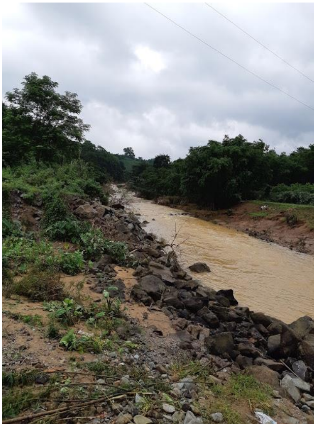
River banks after dam with clear soil erosion and deposition of sediments (left side) due to high river flows during rainy events
