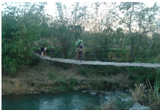
Old Bridge to the nearby hamlet before the project started
