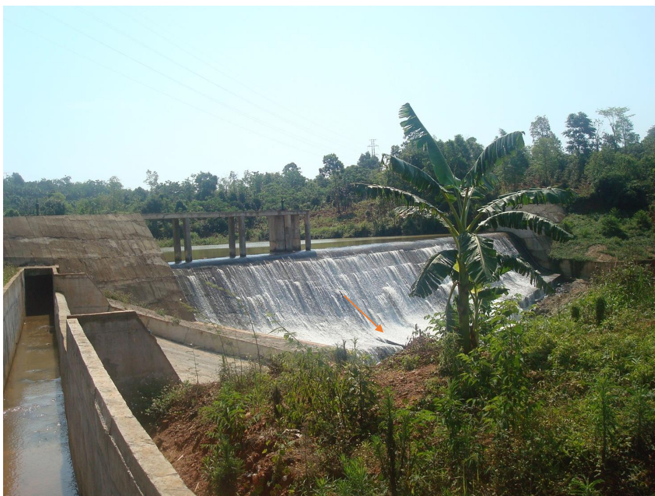
Picture Dam with the sediment flushing opening (red arrow). During rainy season the surplus water flows over dam.
