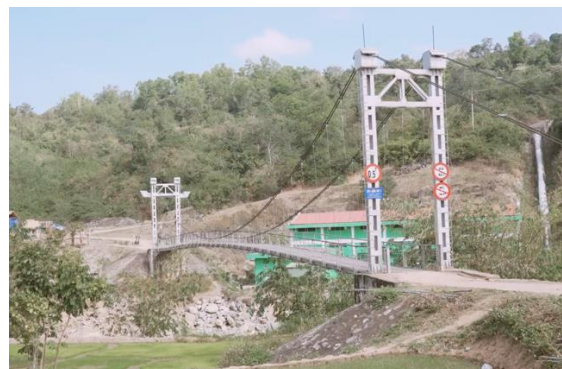
Road and bridge renewed by the project activity
