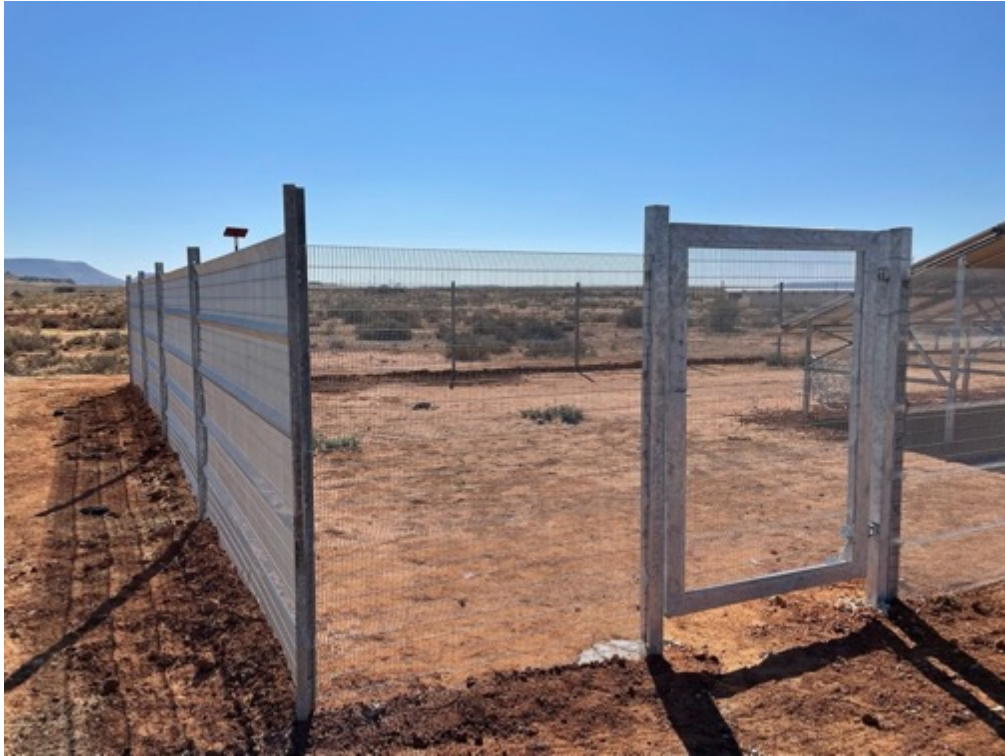
Figure 7 – Photos of re-equipped boreholes (continuation)
