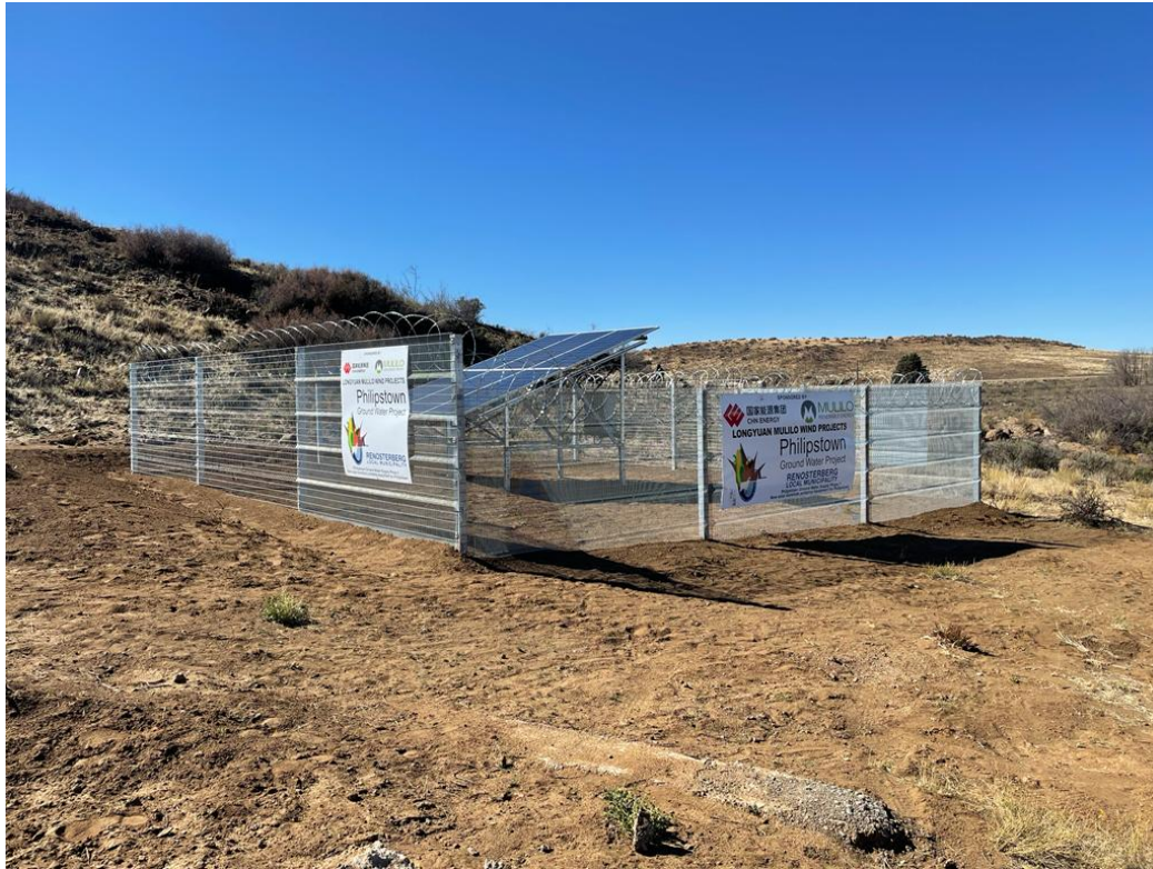
Figure 7 – Photos of re-equipped boreholes (continuation)
