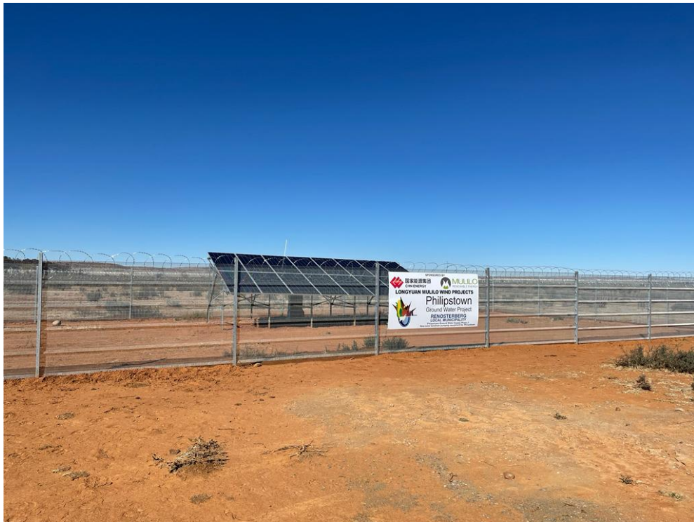
Figure 7 – Photos of re-equipped boreholes (continuation)
