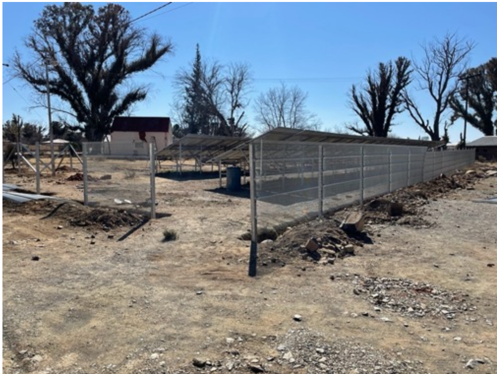
Figure 7 – Photos of re-equipped boreholes
